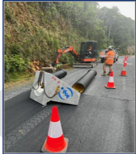
Culvert repair work
