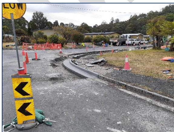
Blackwood Avenue works in progress
