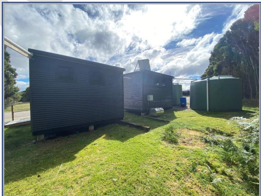
Burbury Toilets external completion
