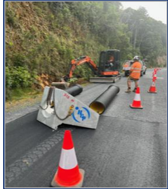
Culvert repair work
